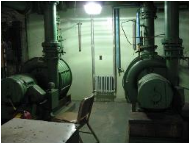
Two of the three raw sewage pumps (10/2007)
