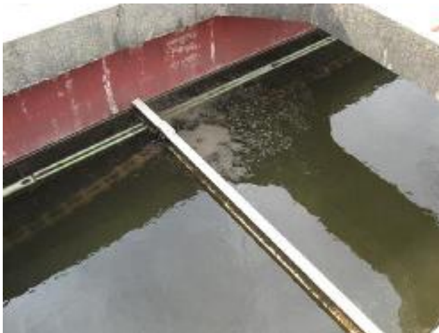
Arm skimming the surface of the clarifier (10/2007)
