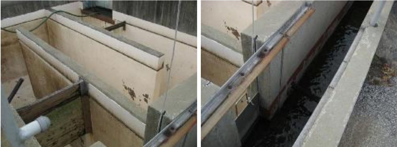
Chlorine chamber ready for winter maintenance (10/2007) Bypass in effect outside of May 15-Oct 15 (10/2007)
