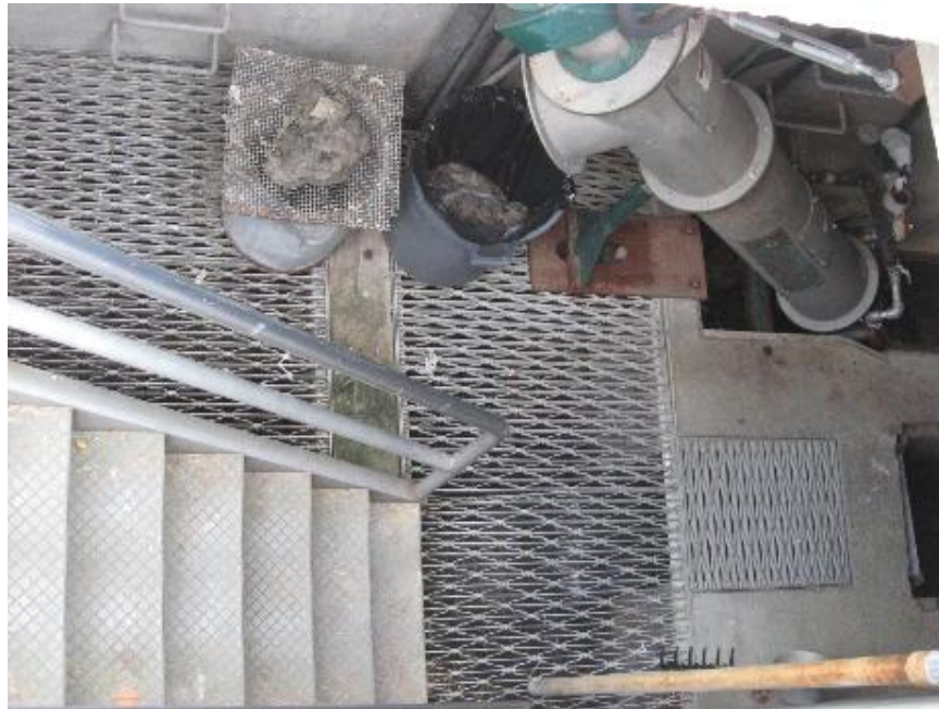
Auger unit currently located in wet well (rags removed manually) (10/2007)
