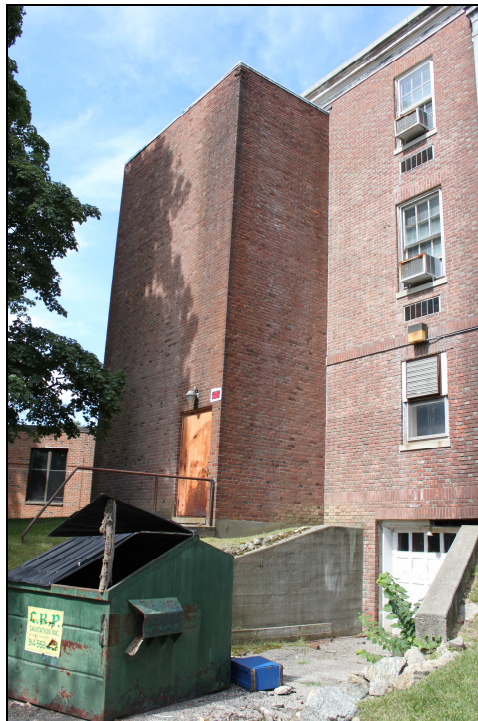
Figure 12: South façade, Timme Wing: At lower right, a rolling door providing access to a partial sub-basement storage and mechanical room that was part of the 1941 design. The exterior fire stair to its right was part of the 1963 hospital complex upgrade.
