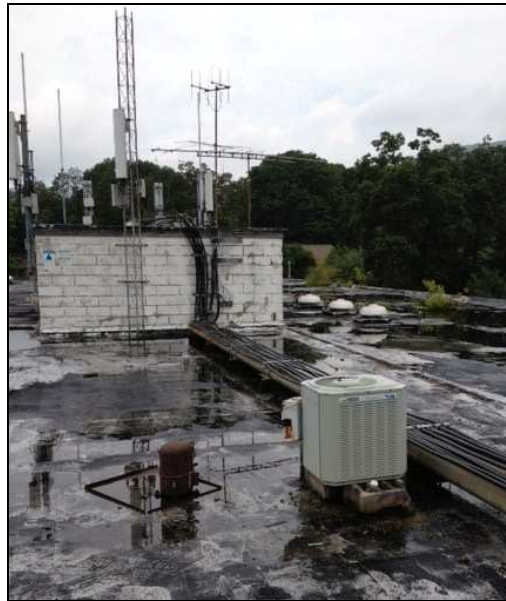
Figure 16: Built-up over the 1925 mass and 1963 addition. The junction of the two structures can be seen in the long diagonal extending just to the right of the concrete mechanicals block.
