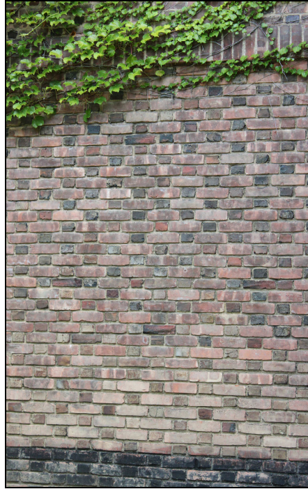
Figure 4: Detail of brick work on the exposed west façade of the 1925 hospital building. Note soldier course at the top of the photo, demarcating the sill line of the above-grade easterly portions of the building.
