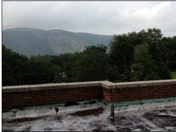
Figure 9: Recessed brick and concrete parapet on roof of the Timme (South) Wing, looking west to Storm King Mountain.
