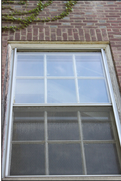
Figure 11: Example of rectangular jack arches above the windows on the 1941 Timme wing.
