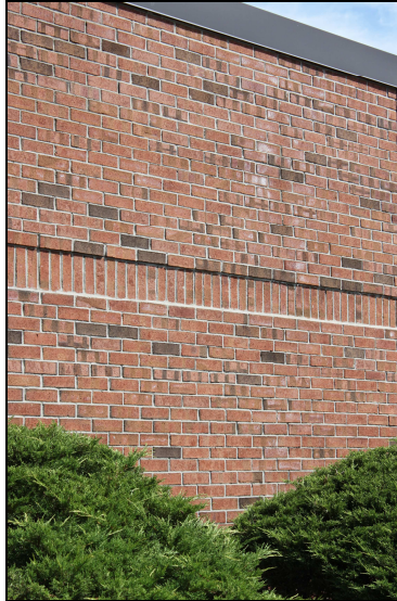
Figure 22: Example of brick work and horizontal banding on the Lahey Pavilion.
