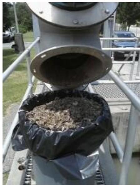
Pictured above is the receptacle for the auger unit. Approximately 3 cubic feet of material is removed from the waste stream every 5 days. If left in the process, the materials reduce the efficiency and lifespan of pumps/motors which can result in higher electrical and repair costs.
