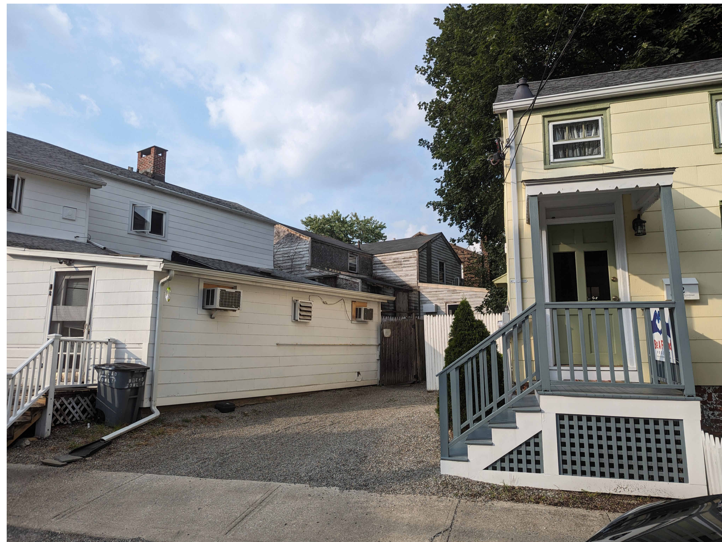
3 EXISTING BACKSIDE OF BUILDING 133 MAIN ST., COLD SPRING, NY
