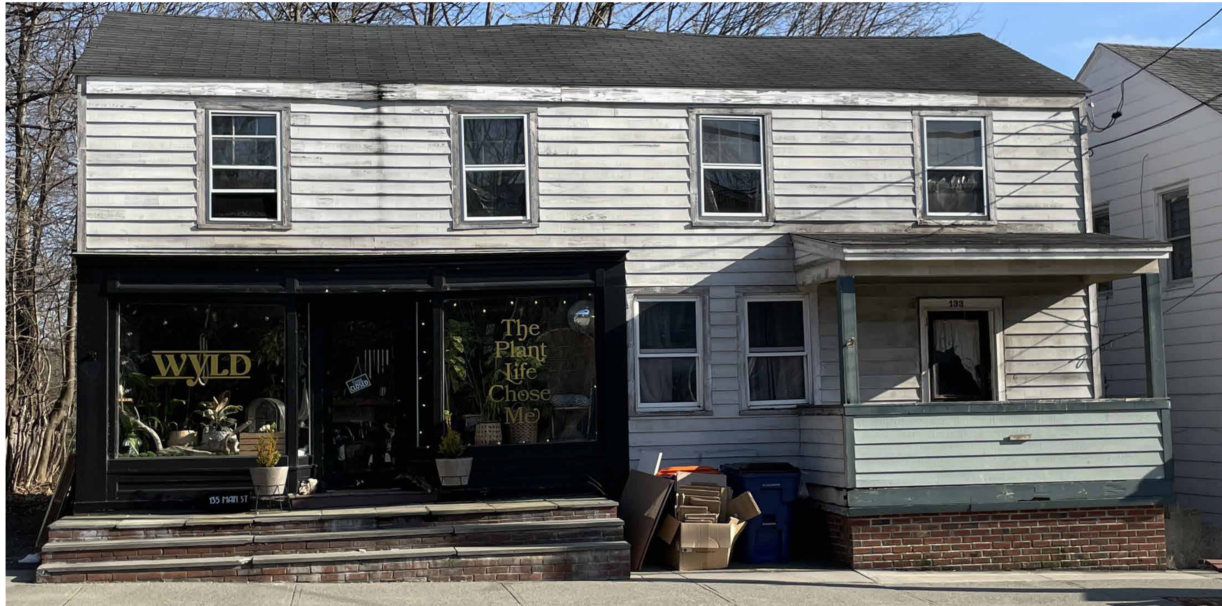
1 EXISTING STOREFRONT OF THE BUILDING 133 MAIN ST., COLD SPRING, NY
