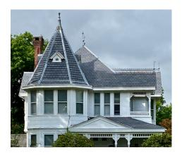
Roofing shall match historic precedent in material, size, exposure, color, and texture. Ornate or rustic patterns are discouraged unless a historic precedent can be documented. Simple shapes and patterns are recommended for asphalt/ fiberglass shingles. Flashing shall be in visually compatible, low contrasting material. Where valleys are deemed character-defining features, they shall be flashed in compatible, traditional materials. Natural roofing materials like slate shall not be painted.
