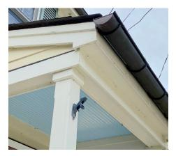
Gutters shall be metal; if natural cooper is used it shall be unpainted. Half round or simple box profiles are preferred; on some 20th Century homes, K-style gutters may be appropriate. Downspouts or leaders shall be the same material as the gutters and shall be positioned to have least impact on publicly visible facades and to achieve maximum water shedding around the building's foundation.
