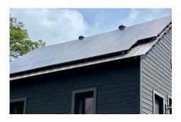
Solar arrays shall be at the same angle as the existing roof and shall be evaluated on a case by case basis. Surface-routed conduits and cables shall be installed in locations with the least visible impact from the public right of way.
